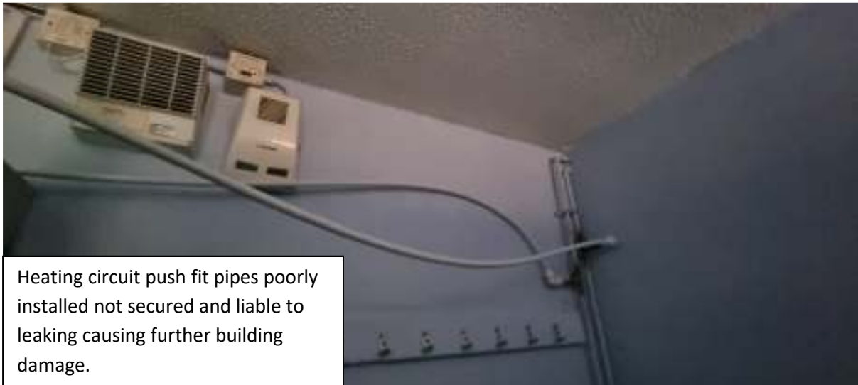
Trunking lid missing, push fit pipe not secured and potential for burst which could drop on someone walking through the door.
