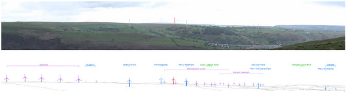
Fig 7. View of the site from the west. Wire line includes operational, consented and application stage turbines.
